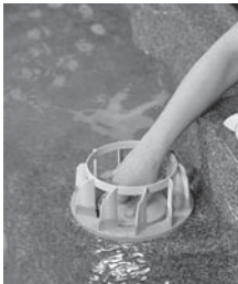
2) Screw filter cartridge in place
