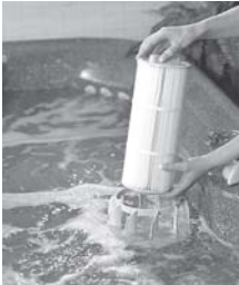
1) Center filter cartridge over canister
