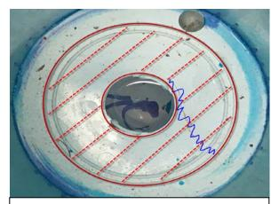
Clean the area in red with the Scotch fiber and soapy water. If there is a crack present, scuff it with the sandpaper for better adhesion Rinse and dry all the area.
