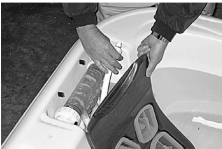
(Figure M-3) Disconnect Air Line Union
