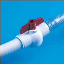
Close drain valve in equipment bay.
