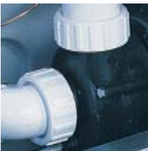
Vent air by slightly opening pump unions.
