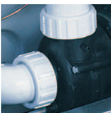
Vent air by slightly opening pump unions.
