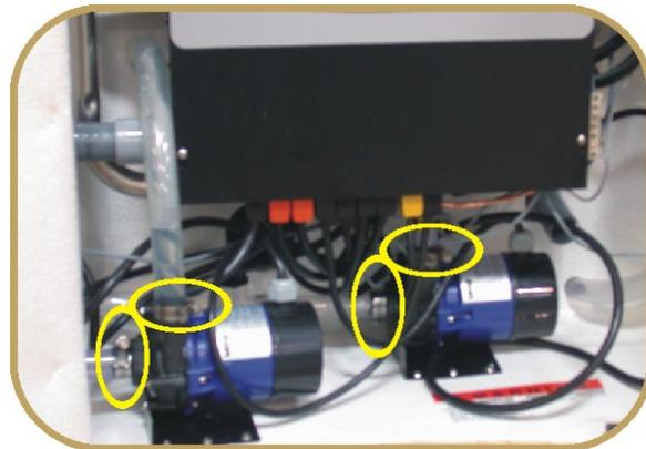
9. Remove the two bleeder valves located near the filters on the top side of the spa. One is located near the skimmer filter (see photo), and the other across the spa near UltraPure™ filter. Removing the bleeders allows air to escape from the pumps when you fill the spa.
