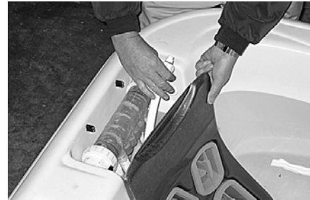
(Figure M-3) Disconnect Air Line Union
