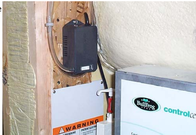
(Figure V) Ozone Sterilizer Location
